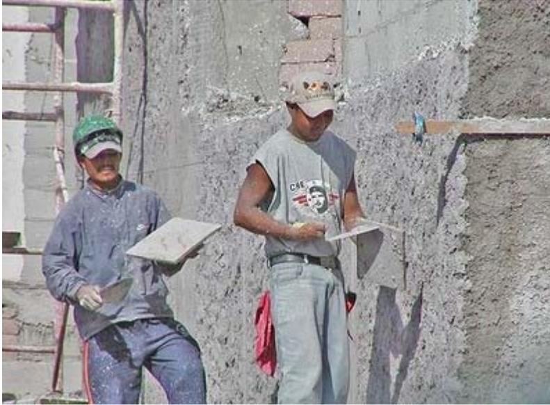
The earth block walls are parged with lime plaster
