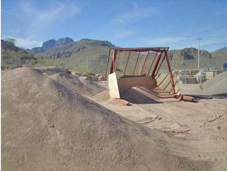
Before making the compressed earth blocks, the clay must be sifted.
