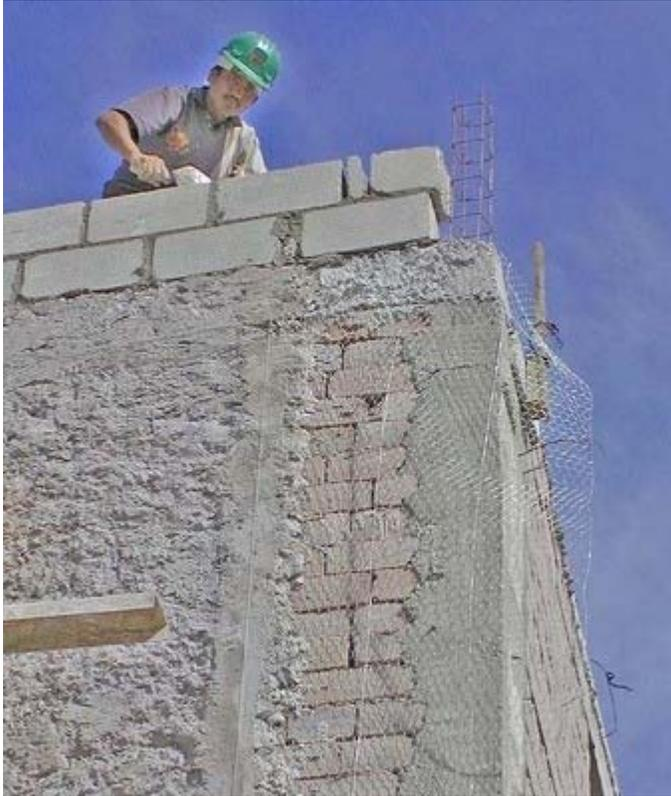
Steel rods and chicken wire reinforce the walls.
