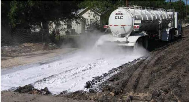
Photo 3: Lime Slurry Placement on Clay Subgrade
