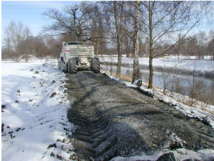
Figure 7: Soil treatment technology with **Proviacal**<sup>®</sup> used during building of flood dike in Hradec Králové.
