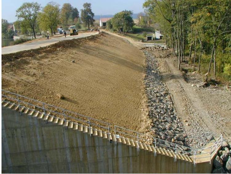
Figure 6: State of Hvězda pond dike after usage of soil treatment technology with **Proviacal**<sup>®</sup>.
