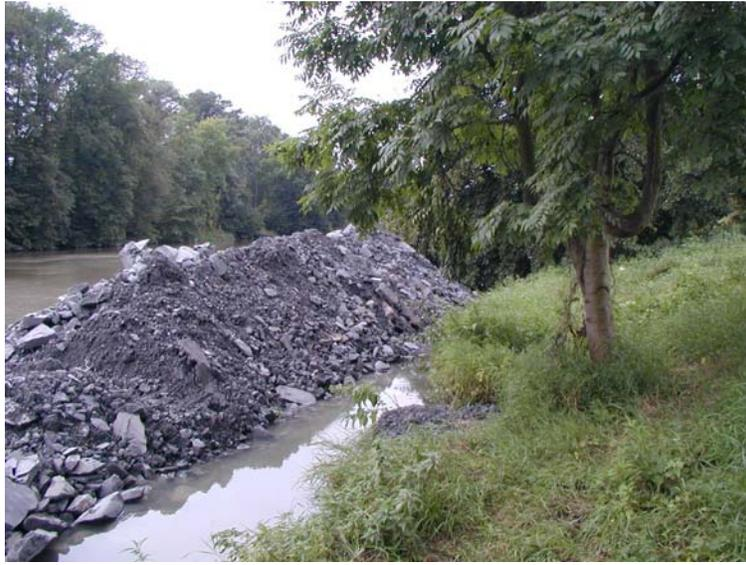
Figure 3: Excavated sediment from Labe river near Pardubice is treated with **Proviacal**<sup>®</sup> and used for flood dikes construction.
