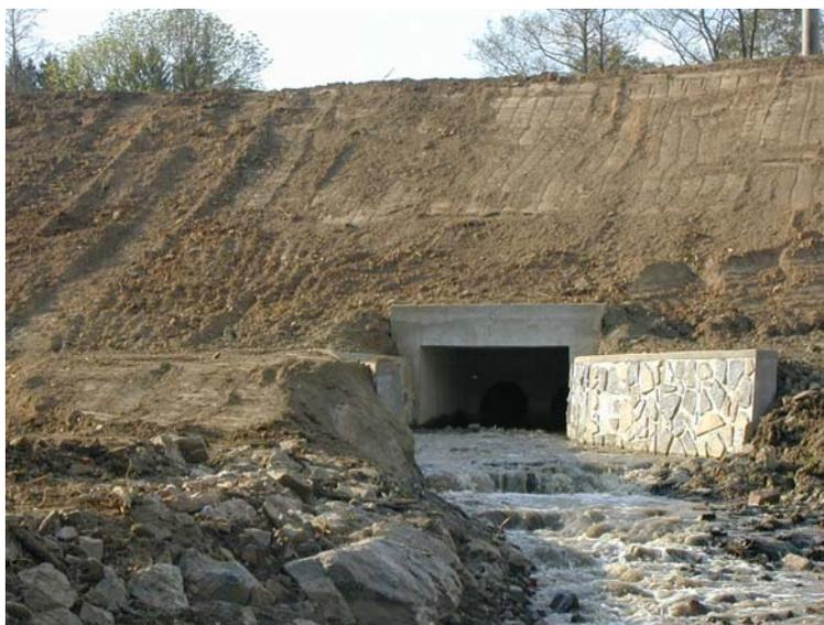
Figure 2: Dike of Chobot pond near Milevsko after reconstruction when soil treatment technology with **Proviacal**<sup>®</sup> was used.
