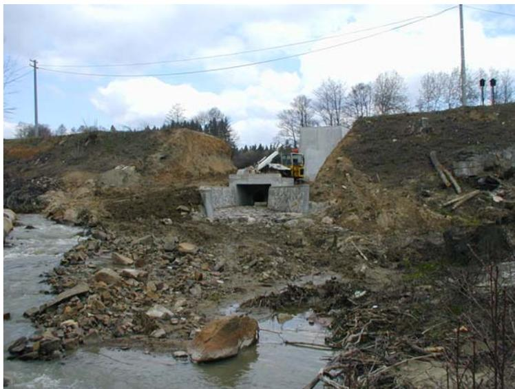
Figure 1: Destroyed dike of Chobot pond near Milevsko during floods in 2002.
