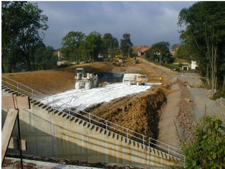
Figure 5: Soil treatment technology with **Proviacal®** used during reconstruction of Hvězda pond dike.
