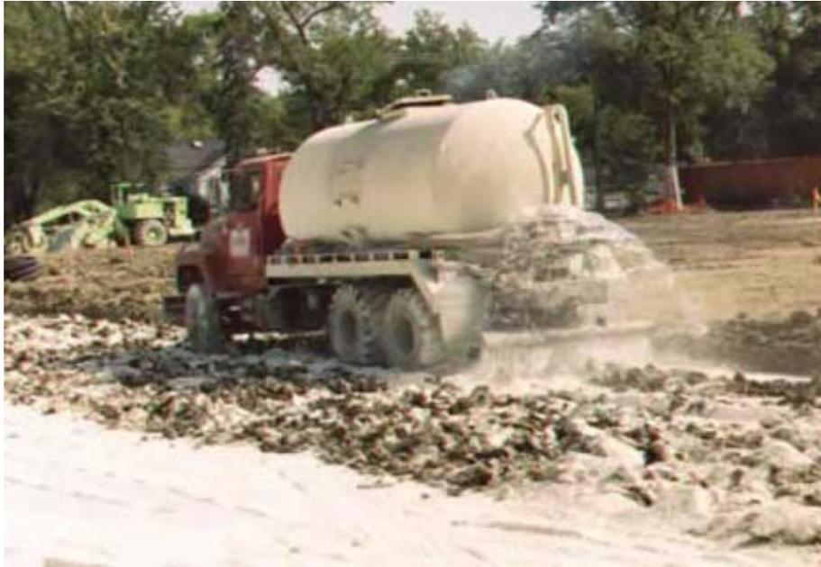
Figure 13: Adding water after dry lime application<sup>5</sup>
