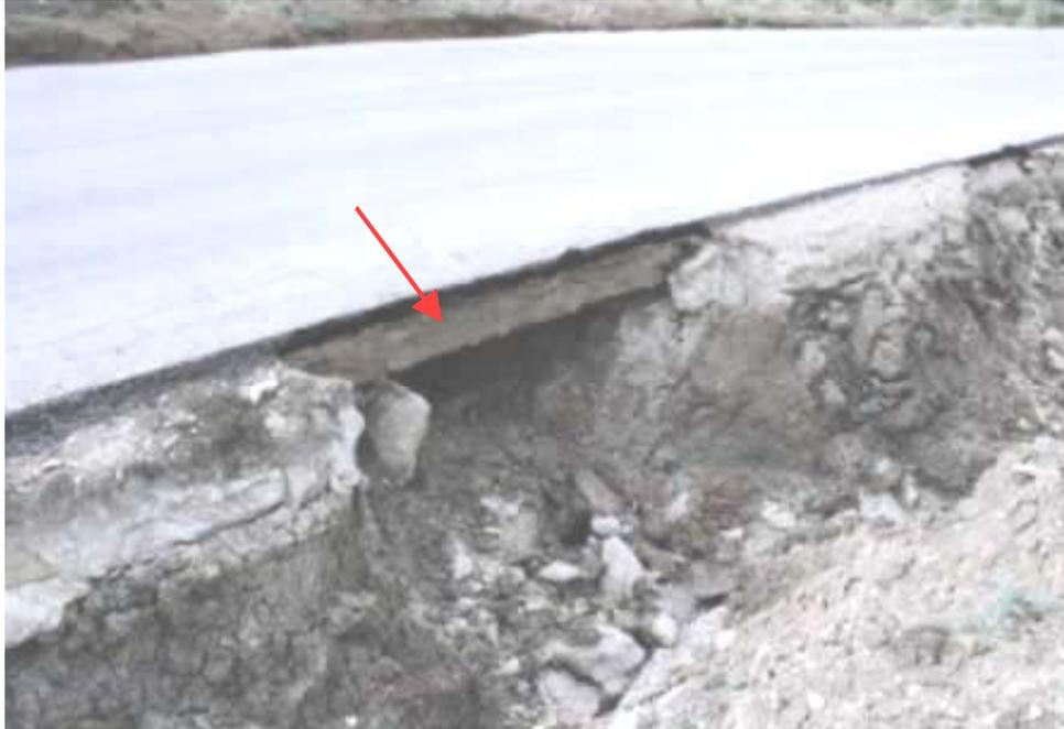
Figure 3: Lime-stabilized layer (see arrow) bridging an erosion failure illustrates strength
