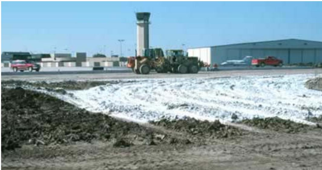
Figure 21: Lime stabilization project at an airport
