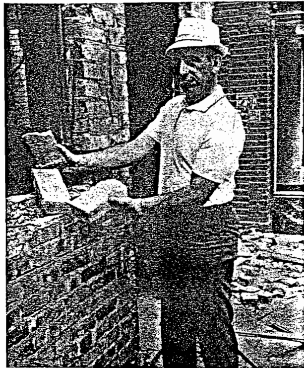
FIG. 10. Wrecking contractor holds sample of old brick-lime mortar from original building in left hand, and backup brick-high cement mortar from modern store front in right hand. Close-up shows intimate contact of old lime mortar, whereas the high cement mortar (held in hand) has "pancaked", breaking clean from the brick.
