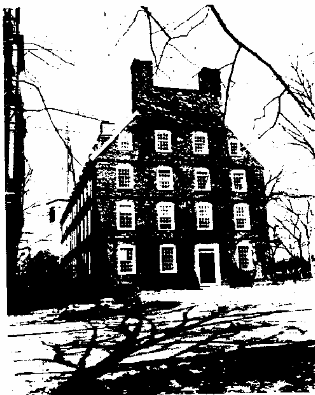
FIG. 1. Massachusetts Hall, Harvard University, built in 1720 with straight lime mortar, has never been tuckpointed.
