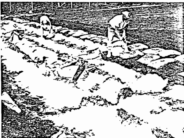
Spreading lime on saturated clay sub-grade of warehouse.
