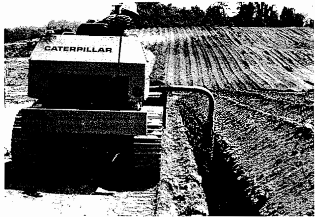
Fig. 1 — Trenching lime-treated dewatered primary sludge on Maryland farm site.
