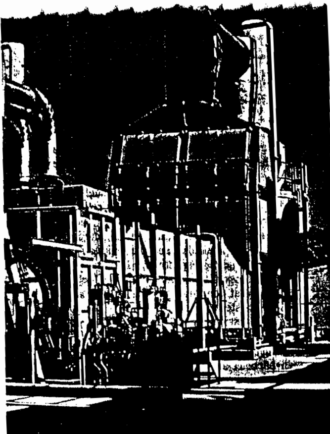
SCR units are in the forefront of NO x -removal efforts.
