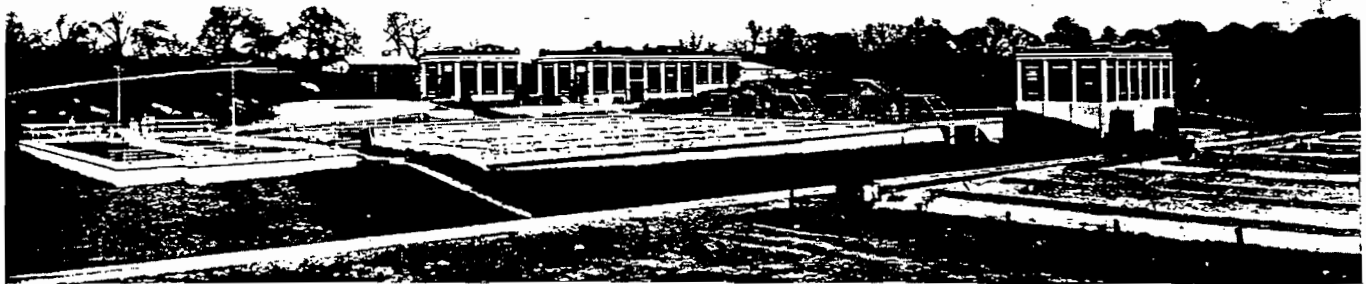
FIG. 1—THE NEW sludge filter building of the Hagerstown sewage-treatment plant and the original sludge-drying beds are at the right. The new office and laboratory and the original service building are in the center background.
