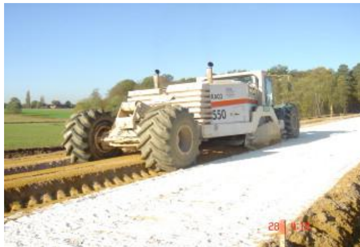
Figure 13: Adding water after dry lime application 5
