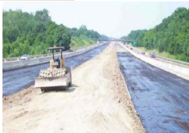
Figure 19: Prime coat emulsion for curing
