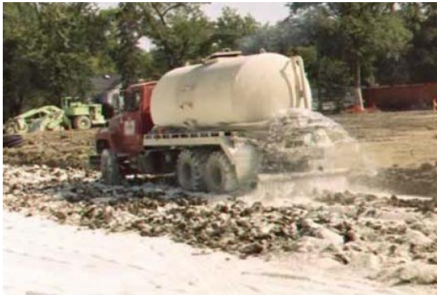
Figure 13: Adding water after dry lime application 5
