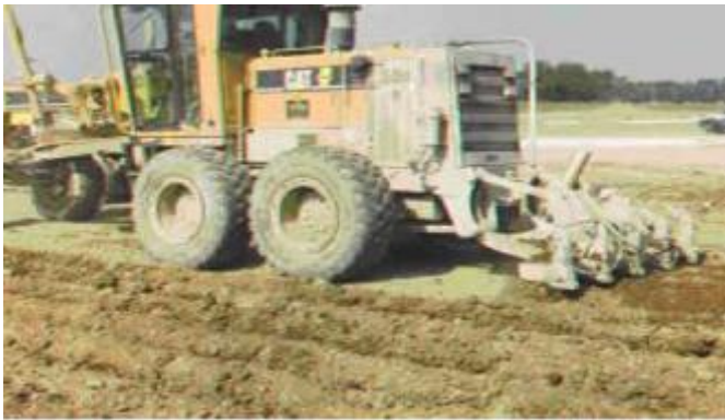
Figure 8: Scarification before lime application
